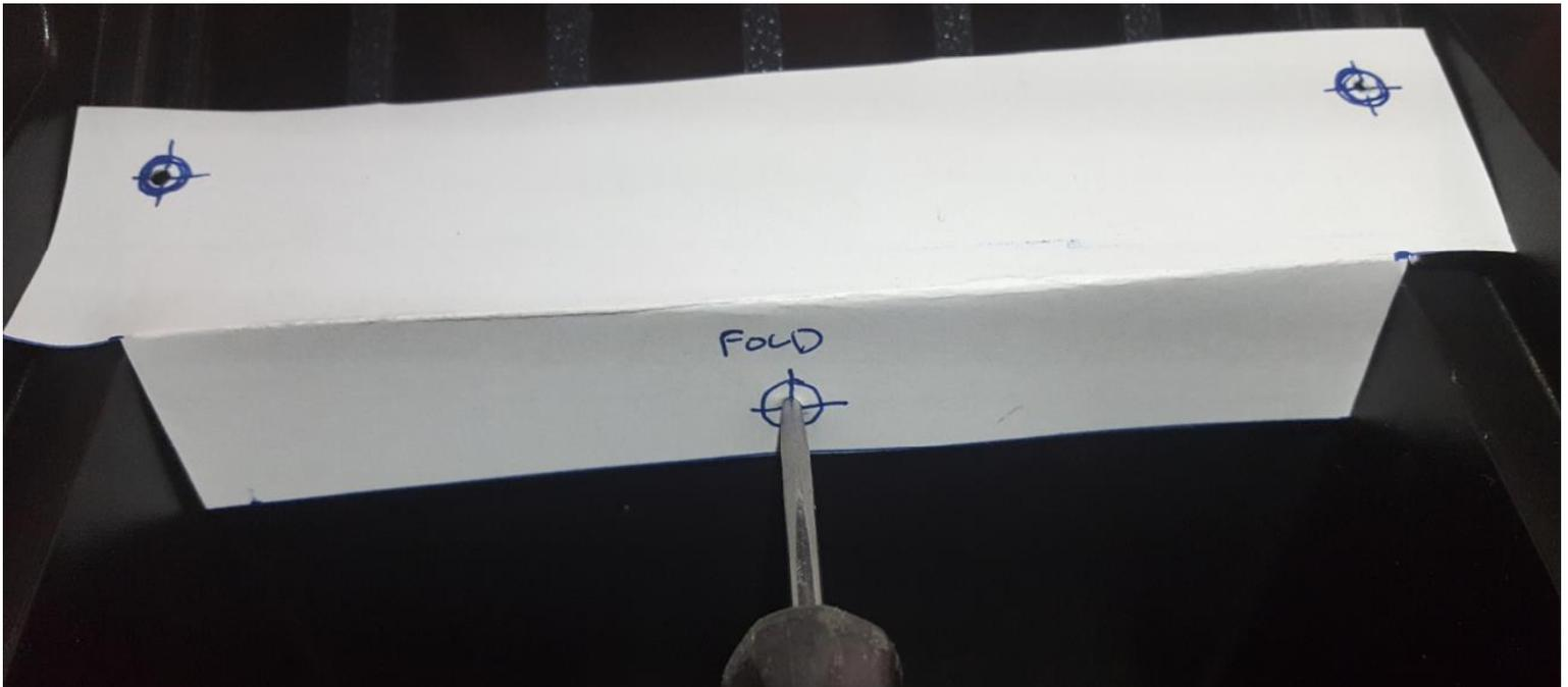
24) Drill all 3 holes with a 1/4" drill bit. Install the faceplate using the 2 shorter black screws provided and tighten. Use the longer black screw provided and install the bottom screw. It helps to use the 1/4 drive Phillips bit, 1/4" socket and 1/4 drive ratchet to install the bottom screw.
